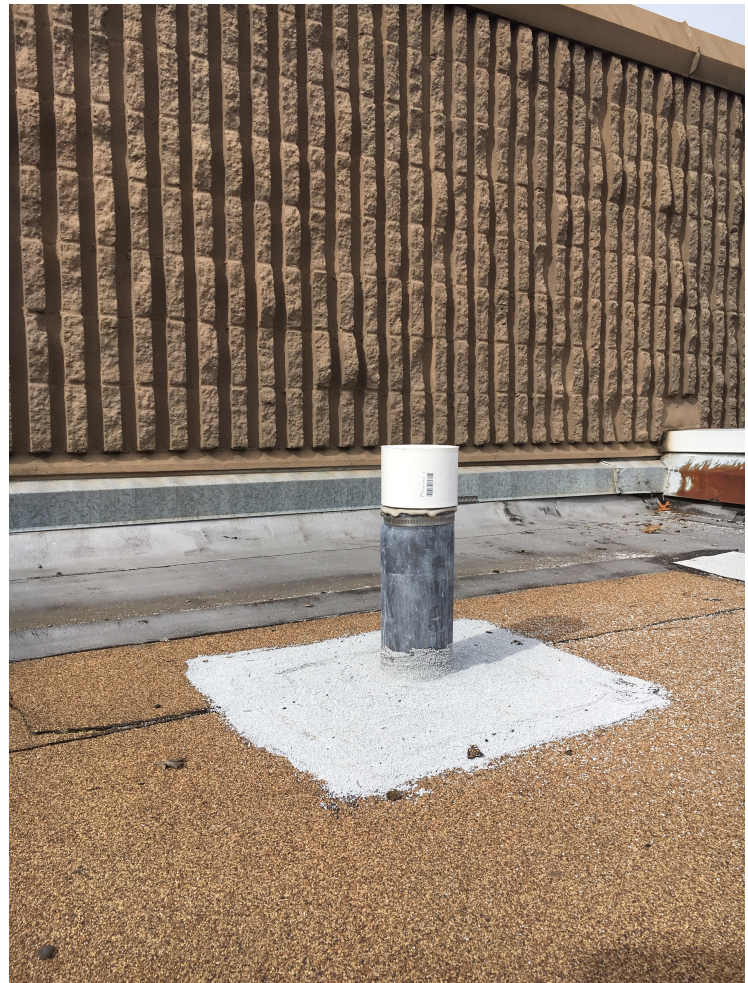
Vent location of system #1
