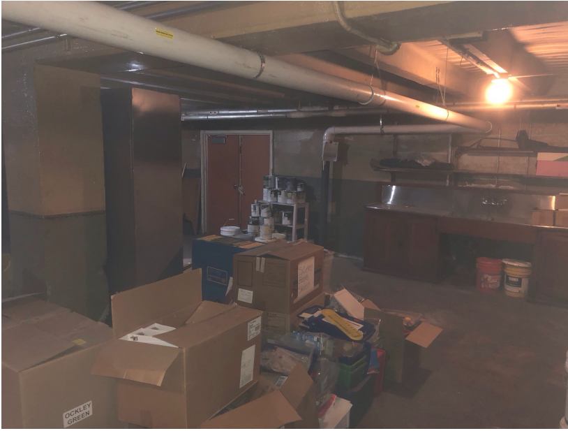
System #2 vent routing in the basement from the suction points and to the western exterior foundation wall. This system is designed to mitigate the Principals Office.
