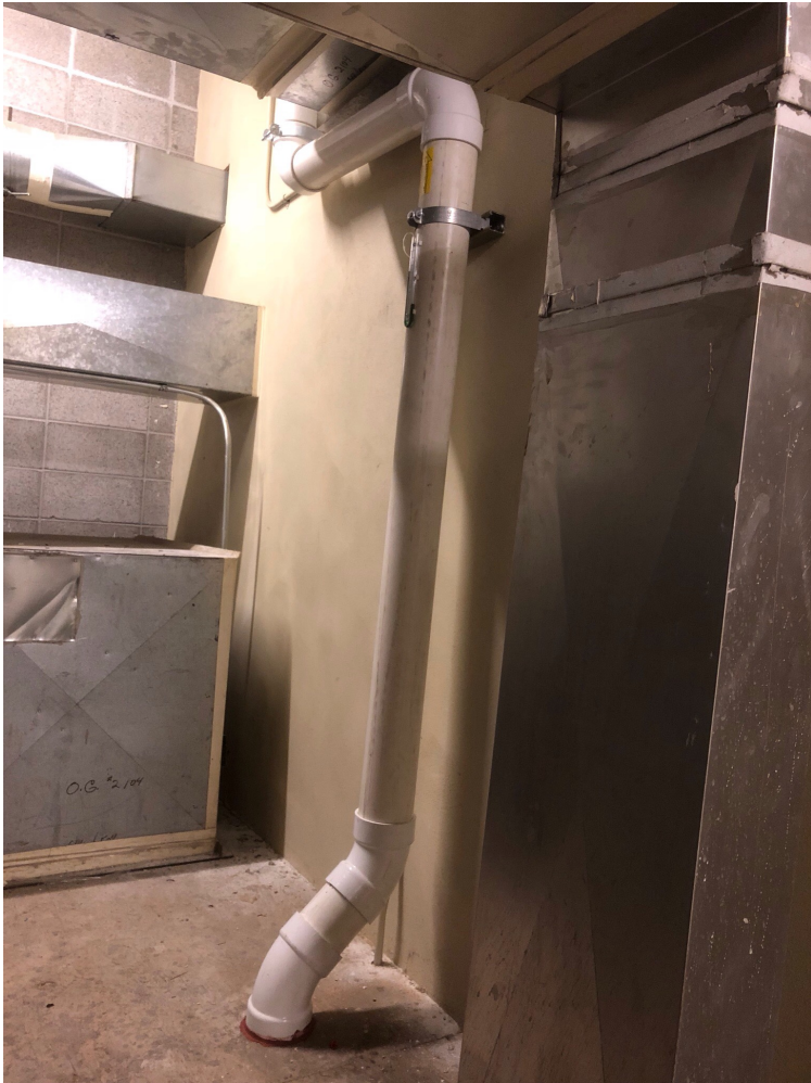
This portion of system #1 is the vent piping continuing from the suction point below in the storage room, into this attic space and up to the mitigation fan.
