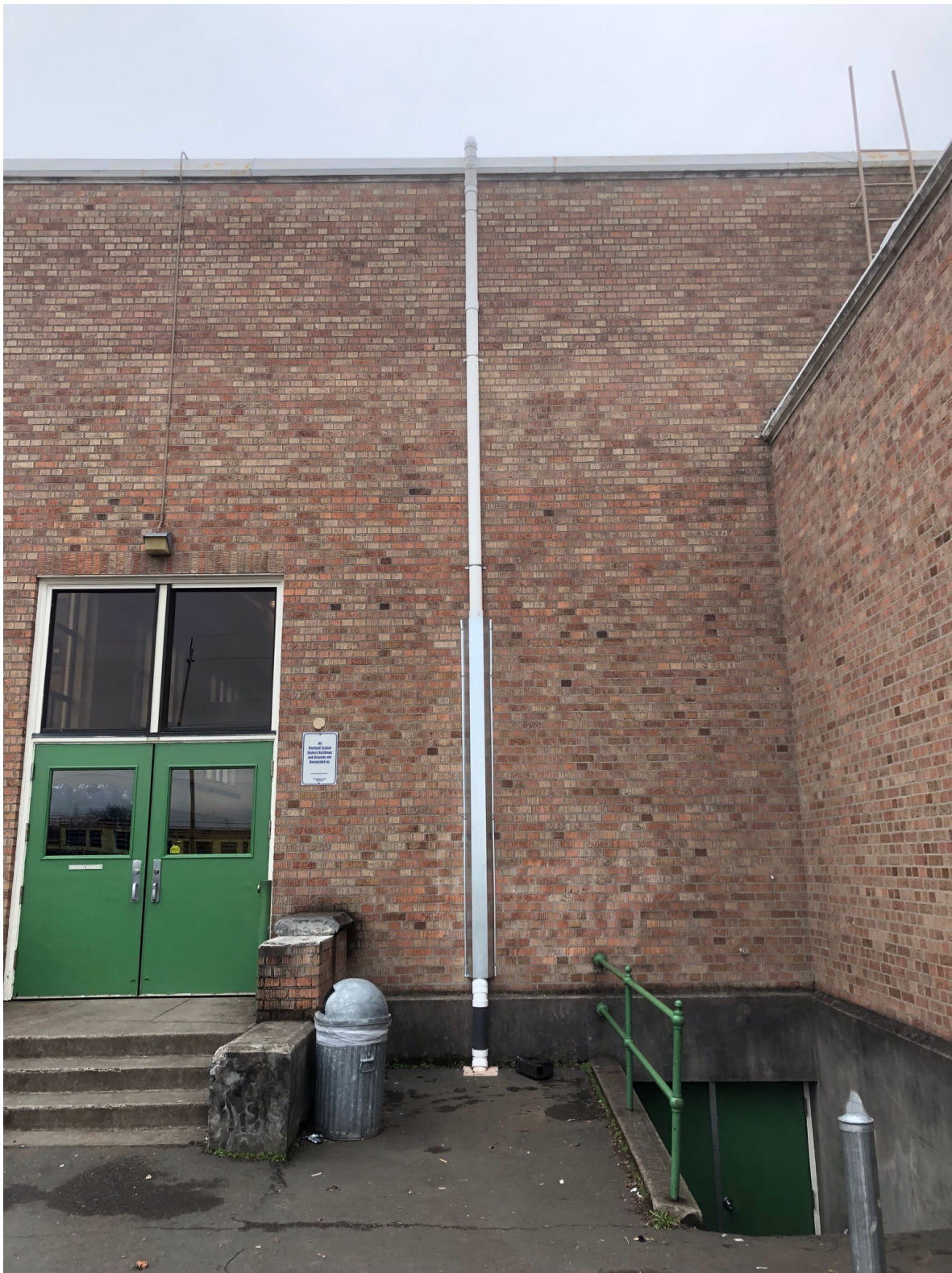
Exterior vent routing to the fan location on the western roof. The exterior vent piping was required to be shrouded to deter climbing.
