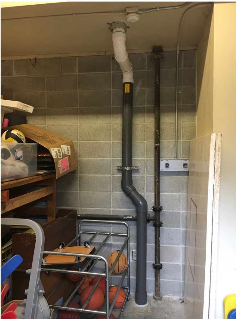
Suction point location in a storage room adjacent to the main gym. Schedule 80 vent piping was used from the floor up to protect against accidental impacts.
